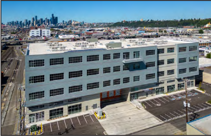
TRACK 6 Seattle, WA 212,516 SF • Four-Stories • 12' - 25' Clear Heights Structural Steel & Concrete Decks • 2.4 Acre Site
