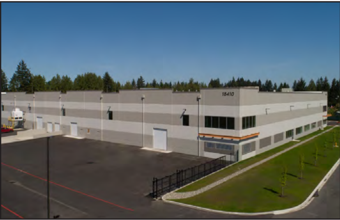
CASTING OPERATIONS Arlington, WA 78,880 SF • 5,500 SF Office • 47,200 SF Manufacturing 16’ Deep Cast-In-Place Pit • 2 Dock-High & 3 At-Grade Doors
