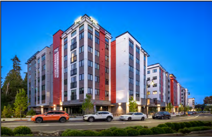
TRAXX Mountlake Terrace, WA 304,877 SF • 6-Stories • 210 Units • Elevated Plazas 14,000 SF Commercial • Extensive Tenant Amenities
