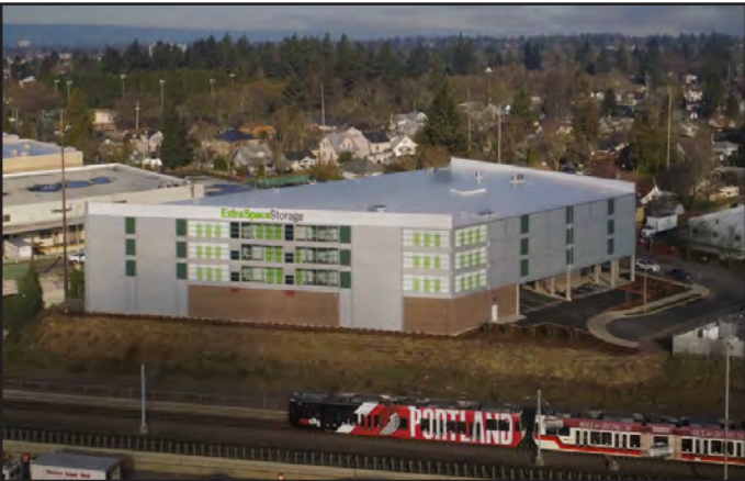
I84 SELF STORAGE Portland, OR 121,220 SF • 4-Stories • 824 Floor Units & 178 Lockers Climate Controlled Units • 50’ CIP Sheer Walls
