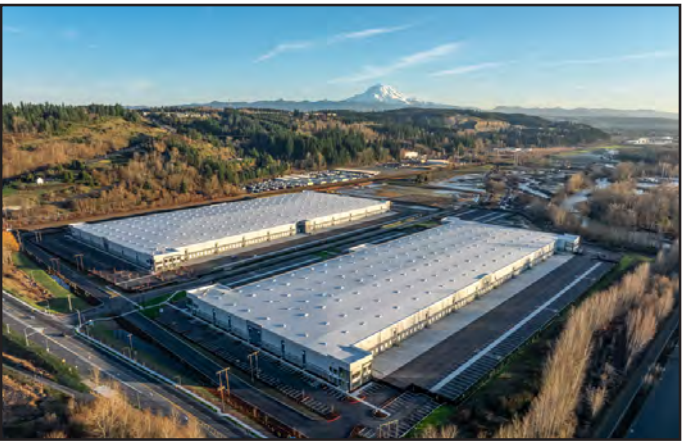
PACIFIC NW LOGISTICS CENTER Sumner, WA 2 Buildings • 476,362 - 705,680 SF • 40' Clear Height 82.6 acre site • 'Sumner Meadows' During Construction
