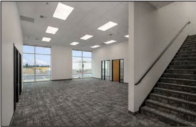
KOWA Frederickson, WA 317,058 SF • 5,942 SF 2-Story Office • HVAC Upgrades Secured Truck Court • 8 Dock Packages
