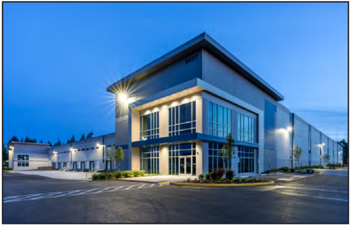
TUMWATER CORPORATE PARK Tumwater, WA 2 Buildings • 199,917 - 199,950 SF • 36' Clear Height Sitework Included Timber Clearing, 4.4 Acre Retention Pond
