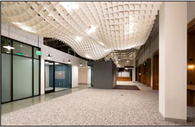
PROLOGIS Seattle, WA 8,000 SF Office Build-Out • 1,740 SF Acousitcal EZO Board 12’ x 30’ Storefront System at Lobby • Alumaglide Systems
