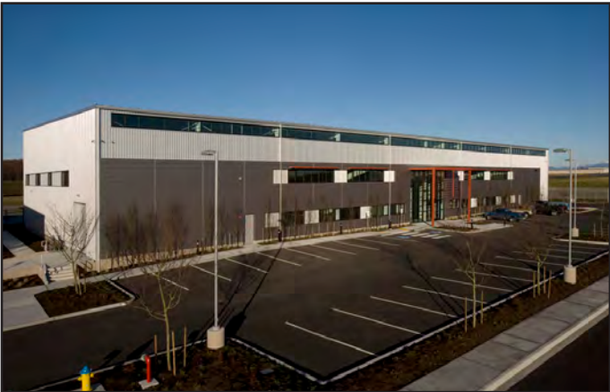
KILO 6 HANGERS Everett, WA 2 Buildings • 16,000 - 27,500 SF • Tip-Up Hangar Doors 1,100’ Taxiway & 1,300’ Access Road • 6 Acre Site
