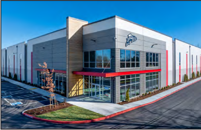
FRANK ALBERT INDUSTRIAL Fife, WA 138,926 SF • 32' Clear Height • 1,000 LF New City Road Puyallup Tribe of Indians Property • 10.58 Acre Site
