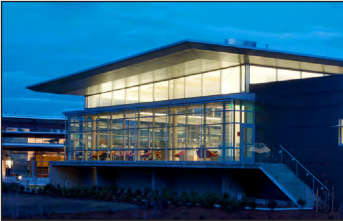
SAMMAMISH LIBRARY Sammamish, WA 20,000 SF • 6’ Gas Fireplace • Stained Concrete Floors Custom Casework • Radiant Heating & Cooling • LEED Gold
