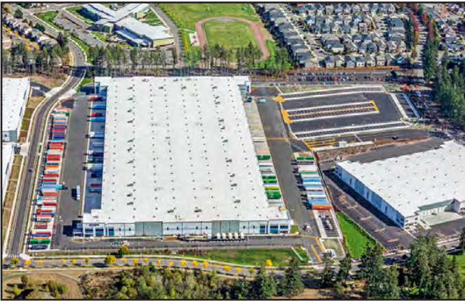
OLM1 Lacey, WA 510,000 SF • 27,000 SF Office Build-Out • MEP Upgrades 133 Dock Packages • New 7.4 Acre Trailer Yard
