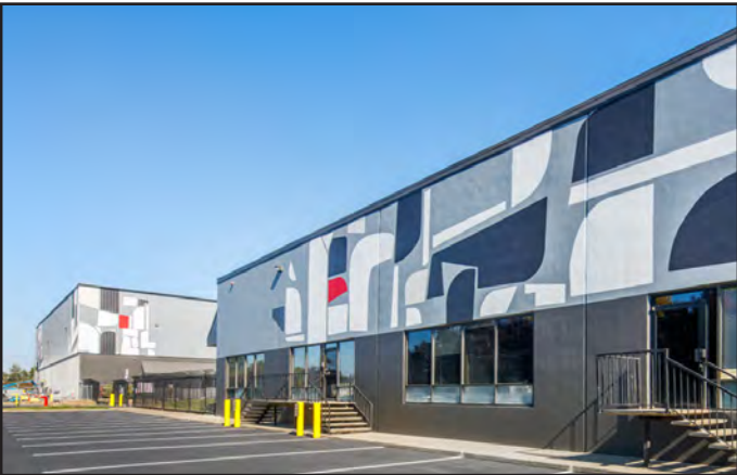
LIFT LOGISTICS RENOVATIONS Kent, WA Interior & Exterior Renovations • 182,000 - 207,744 SF MEP System Upgrades • Utility Upgrades • Site Improvements
