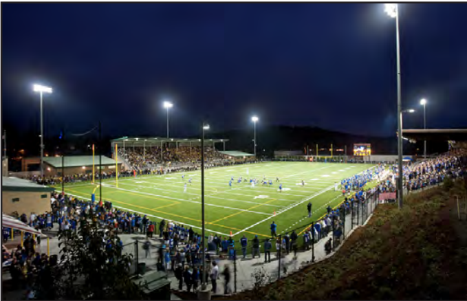
POP KEENEY STADIUM RENOVATION Bothell, WA New Visitors Grandstand • Lighting & Parking Lot Upgrades New Concession Stand, Locker Rooms & Restroom Facilities
