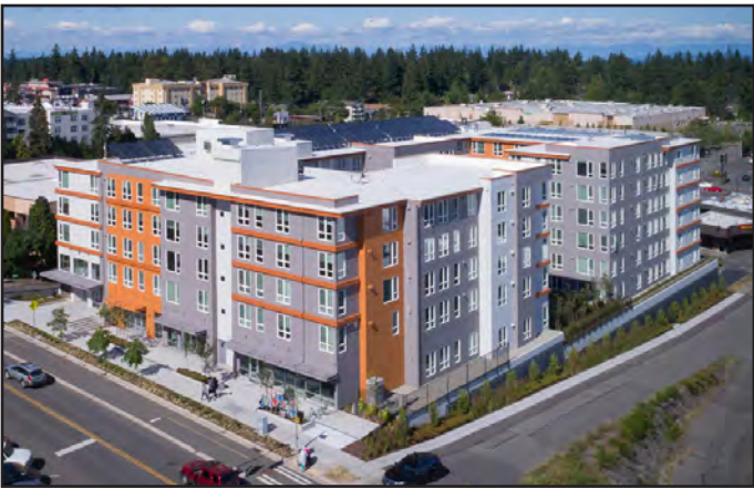
LINDEN FLATS Seattle, WA 201,617 SF • 7-Stories • 170 Income Qualified Units Solar-Thermal Water Preheating & Photovoltaic Systems
