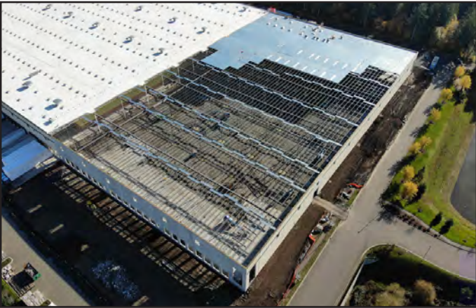
ULINE S6 EXPANSION Lacey, WA 189,810 SF Expansion to 810,988 SF Distribution Center 1,682 SF Office • Re-Utilized 24 Tilt Panels • 26 Dock Doors
