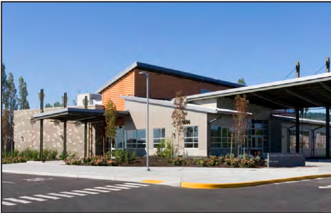
NCTA MARINE TECH CENTER Anacortes, WA 18,189 SF • Classrooms & Labs • Geo-Thermal Heating Structural Steel & CMU • 213 Solar Panels with 48W Output
