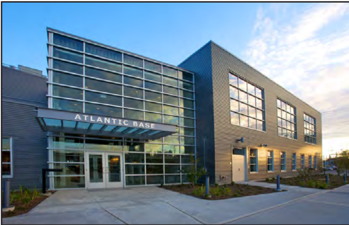
ATLANTIC CENTRAL OPERATIONS Seattle, WA 44,345 SF • 2-Stories • Build-Out • Terrazo Flooring Suspended Glass Flooring • LEED Gold
