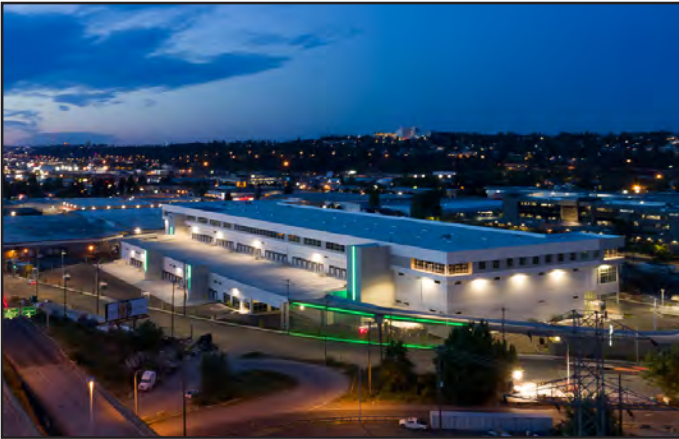
GEORGETOWN CROSSROADS Seattle, WA 590,000 SF • LEED Gold • Full Size Truck Ramp to L2 16' - 28' Clear Height • Four Story Parking Structure
