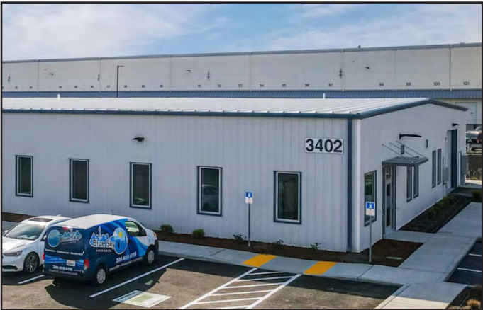
PORTSIDE 55 EAST Tacoma, WA 10,200 SF • Pre-Manufactured Metal Building 3.54 Acre Site
