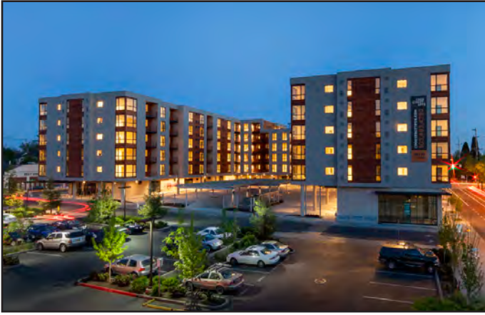
COOK STREET APARTMENTS Portland, OR 240,041 SF • 6-Stories • 206 Units Below & At Grade Parking • 15,000 SF Commercial
