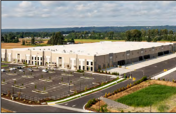
PEPSICO Marysville, WA 307,493 SF • 17,321 SF Office • 10,382 SF Maintenance Shop 56 Dock-High, On-Grade & Fleet Dock Doors • 36’ Clear Height
