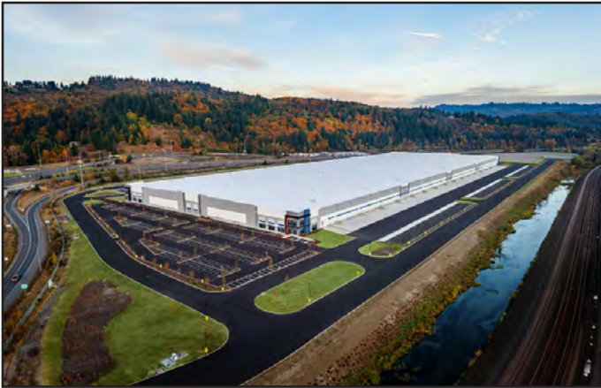
MID I-5 INDUSTRIAL Kelso, WA 1,185,327 SF • 40' Clear Height • 116 Acre Site Site Required 59,000 Deep Dynamic Compaction Drops
